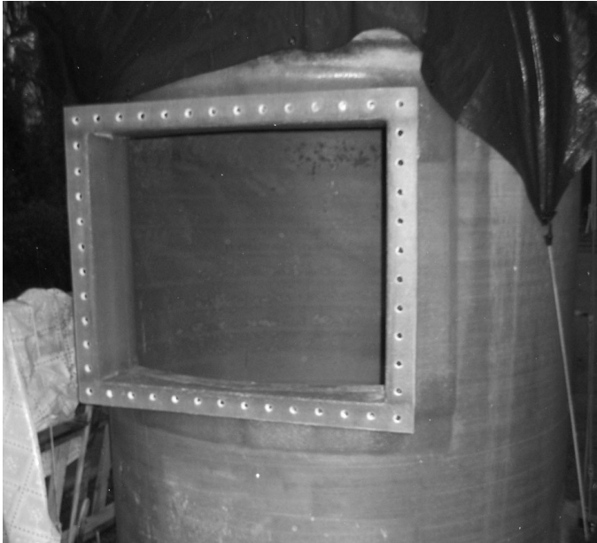
The window frame installed with all bolt holes bored.
