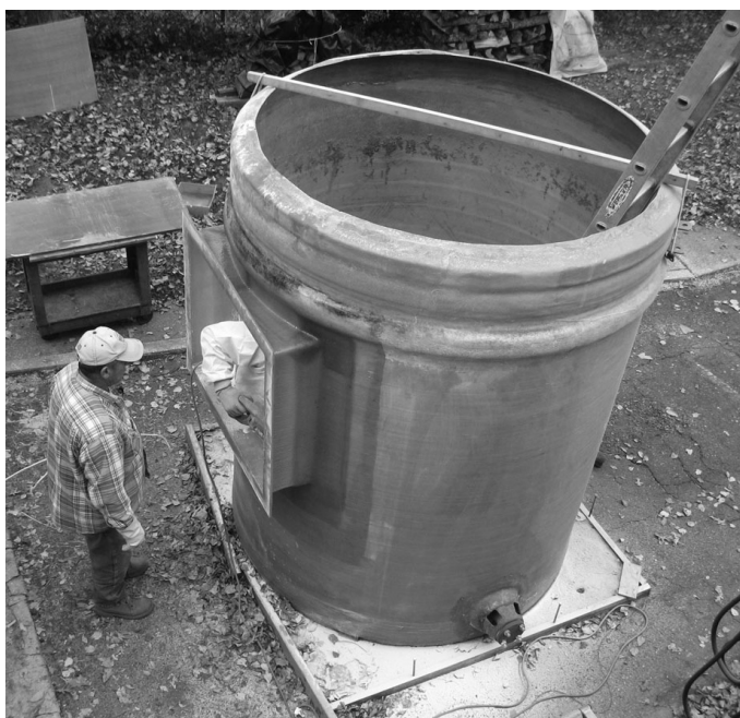
Installing the window frame.
