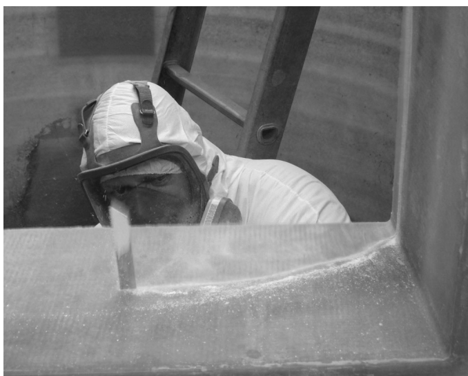
Trimming the frame to the shape of the tank.
