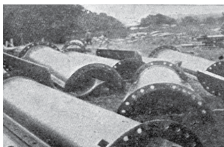
Steel semi-cylinders for the Marconi tubular mast
